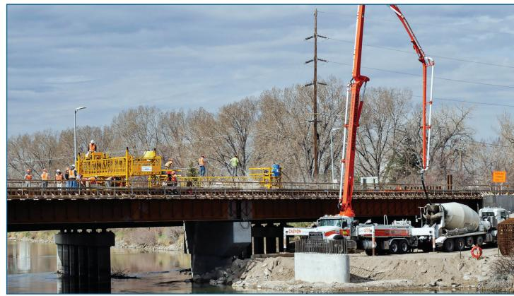
Workers with general contractor Ames Construction keep the concrete flowing April 24 as they pour the concrete deck atop the northbound I-25 bridge over the North Platte River in Casper.
