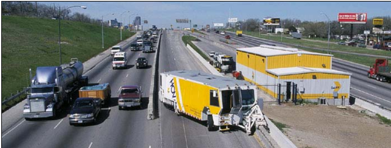
Exhibit 6b: Movable Barrier System in Use, I-30 Dallas, Texas
